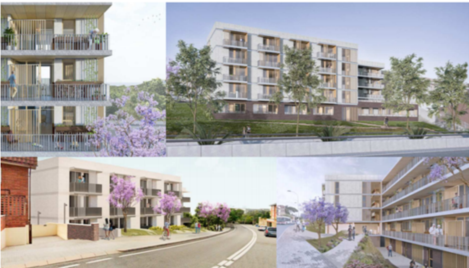
Figure 1. Render of the 34 social buildings destined for the elderly on Carretera de Sant Cugat. Source: Ajuntament de Barcelona (2020)
