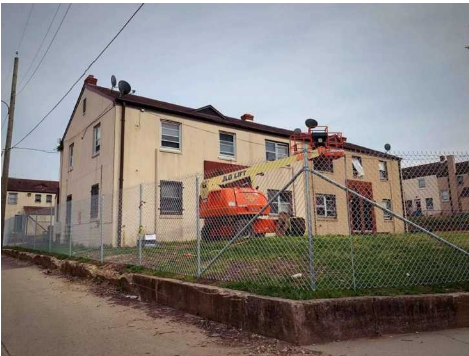
The changing urban fabric of Anacostia, Washington, DC - demolition of Barry Farms public housing development.
